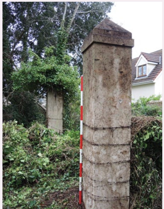
Concrete entrance posts wrapped in barbed wire.
