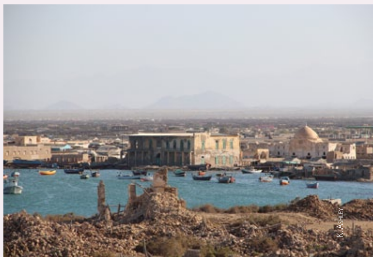
Suakin School (centre) in its setting before reconstruction, as viewed from the Island Town.
