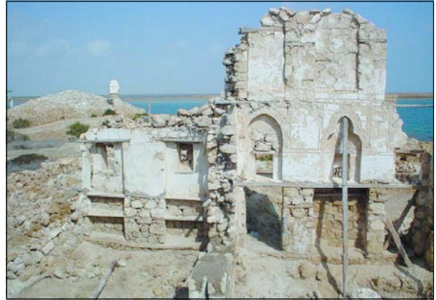
Remains of walling of Khorshid Effendi House, showing decorative plasterwork (Photo: M. Mallinson.)
