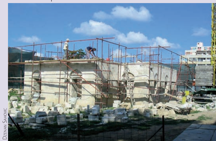
Rebuilding of the Ferhadija Mosque in Banja Luka, northwestern Bosnia.
