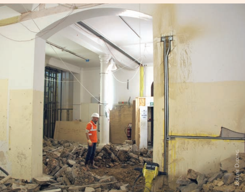
Archaeology of the Museum's archaeology gallery: digging out the old floor. No archaeological finds were made in these many tonnes of concrete!
